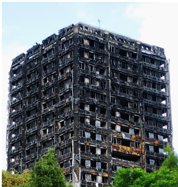
Grenfell Tower 14 juni 2017
